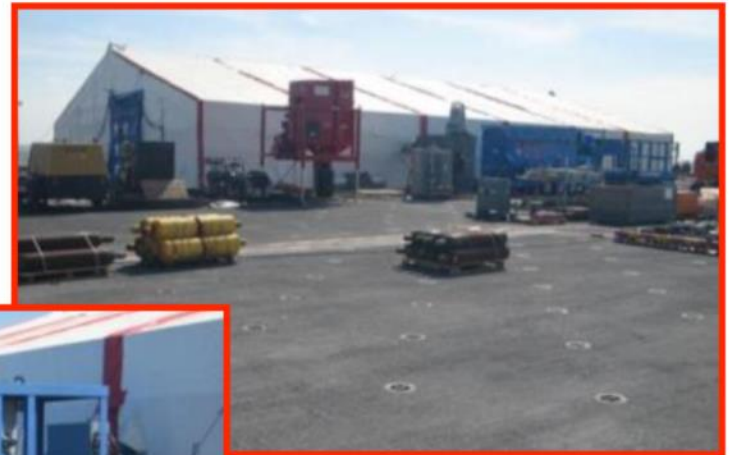
Overview of Enclosure
